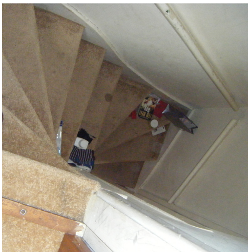
3 Staircase looking down from top floor landing
