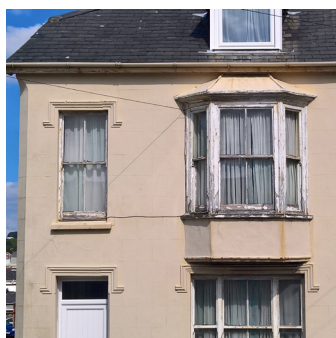
1 Front of the property showing the poor condition of the original windows
