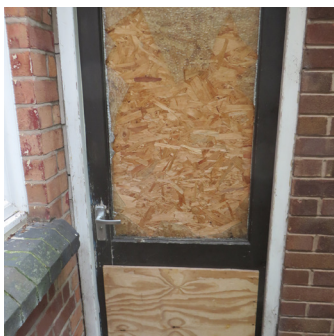
3 Rear door boarded over due to broken glass panel
