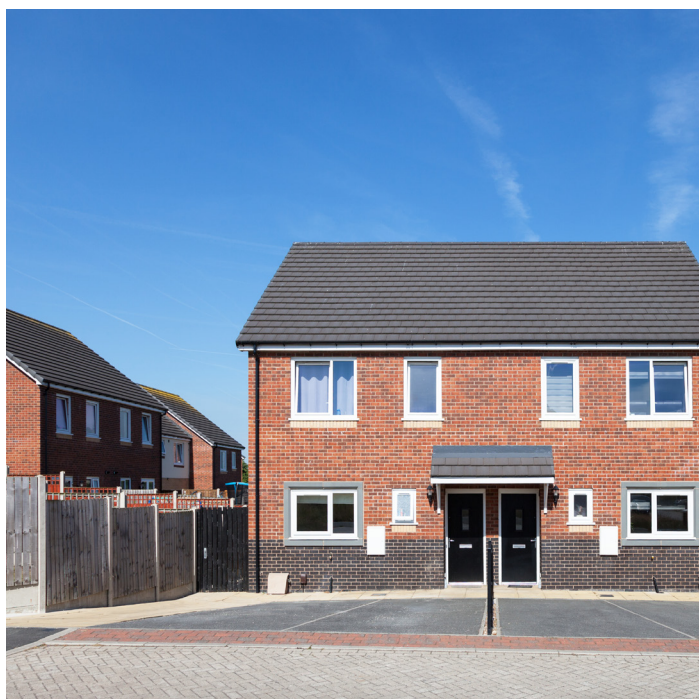
1 Front exterior view of property
