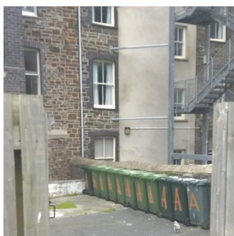
2 Rear elevation of property
