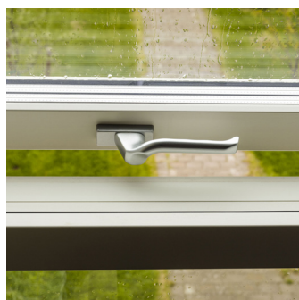
2 Window open demonstrating restriction of less than 100mm
