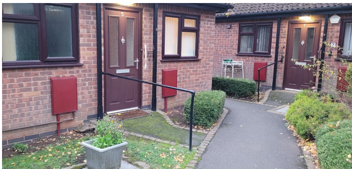
1 Front of the property showing the distance of the front door to the footpath
