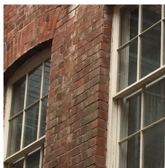
3 Close up of single glazed sash window in living room
