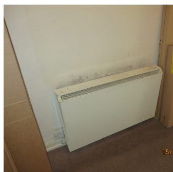
2 Electric storage heater in living room with mould growth to wall
