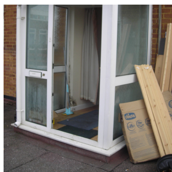
3 Entrance porch and flat roof exterior
