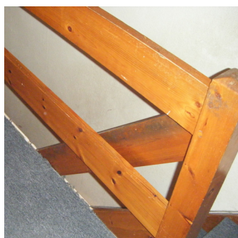
2 First floor landing balustrade
