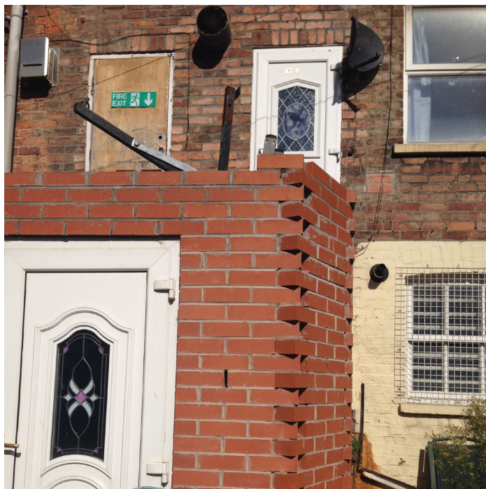
3 Rear flat roof
