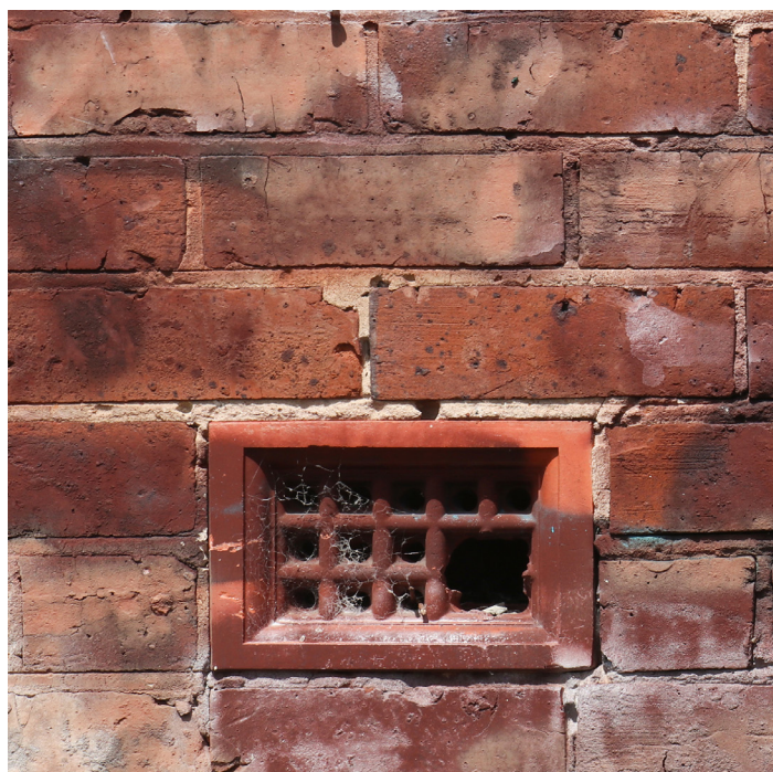
3 One of the broken airbricks at rear of the property
