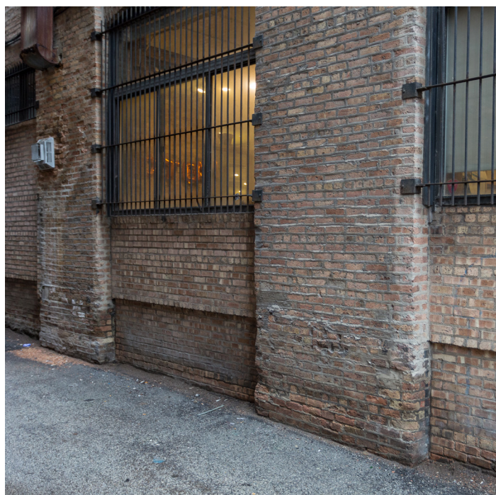
1 Exterior view of barred windows in shade
