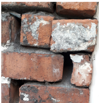
4 Damaged brickwork
